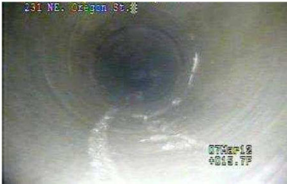
Camera shot of repaired line.
