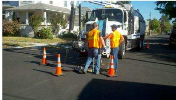
McMinnville Conveyance System Maintenance Crew doing maintenance inspections of the City's sewer lines.
