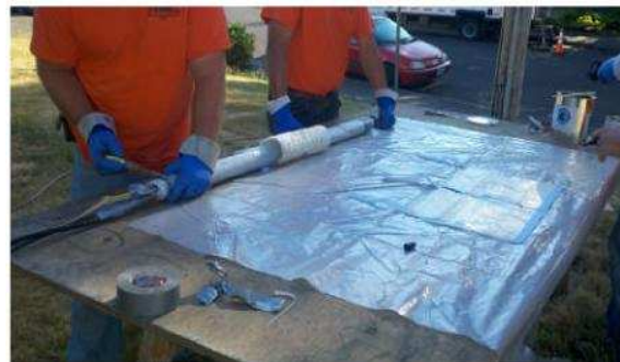
McMinnville crew preparing the carrier and liner for insertion into line.
